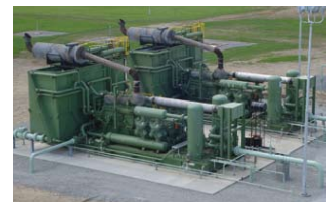
Final Location: Fast-track project, completed in just five months.
